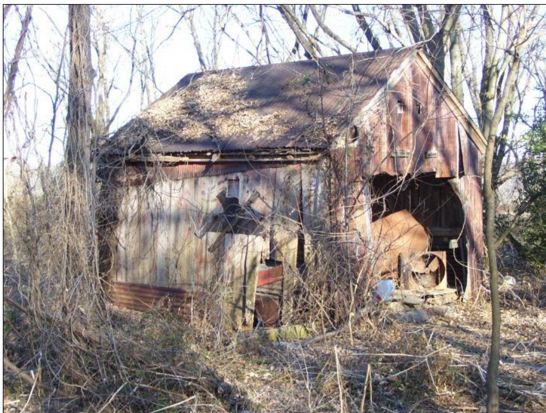
Figure 11: Standing Shed, Structure 6.
